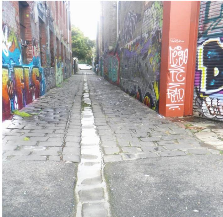
These tall warehouse buildings were built about in 1840 in Melbourne. Their huge slate roofs collect lots of rain and channel it into a few downpipes. These pour fast flowing water into little lanes like this one. Eventually the water is channeled into drains under the pavement
