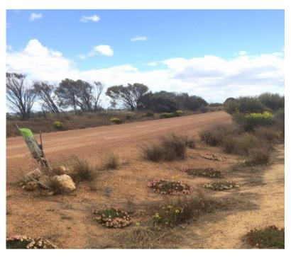
Why is the level of the road above the level of the adjoining countryside? To allow rain water to drain away
