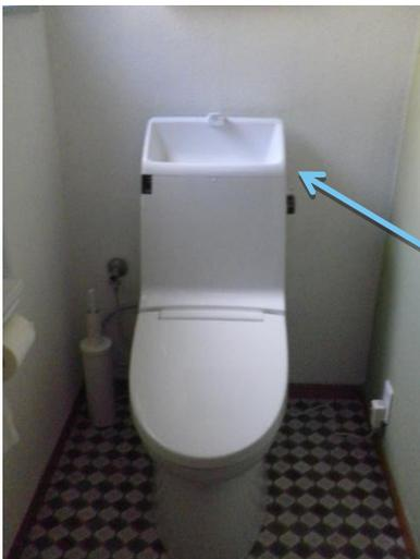
4. Toilets should be dual flush to minimize water use. In some Japanese schools' "intelligent" toilets are installed. There the water used to wash your hands is held in a basin at the top of the toilet then channeled down to flush the toilet too! The Water Corporation has a lovely video of a singing toilet for National Toilet Day.
