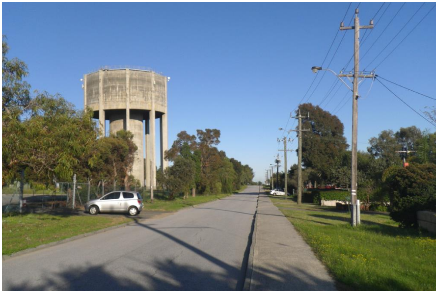
Gravity feed water tank that increases water pressure for the Perth suburb of Coolbellup.
