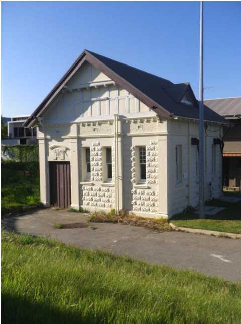
Small pumping station in South Fremantle (built 1934 - now unused)
