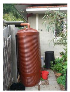
Water can be collected from house roofs and downpipes and directed into rainwater tanks for storage. It is filtered to remove any dead leaves or material from the roof and to prevent birds, frogs and lizards from entering. Does your house have a rainwater tank?
