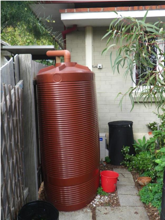
Rainwater can be collected directly from house roofs and downpipes and directed into rainwater tanks for storage. Water is filtered before entering the tank to remove any dead leaves or material from the roof and to prevent birds, frogs and lizards from entering. These tanks also often have screens to prevent insects such as mosquitos and flies from contaminating water. When properly maintained this water is good for most household and garden purposes.
